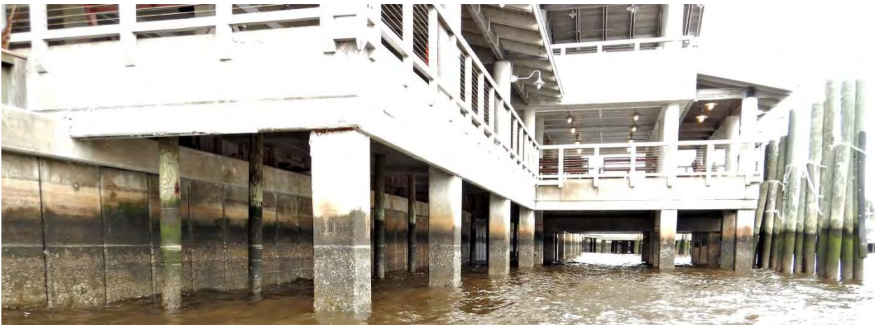
End view of concrete support piles, timber fender piles (right), and adjacent concrete bulkhead (left)
