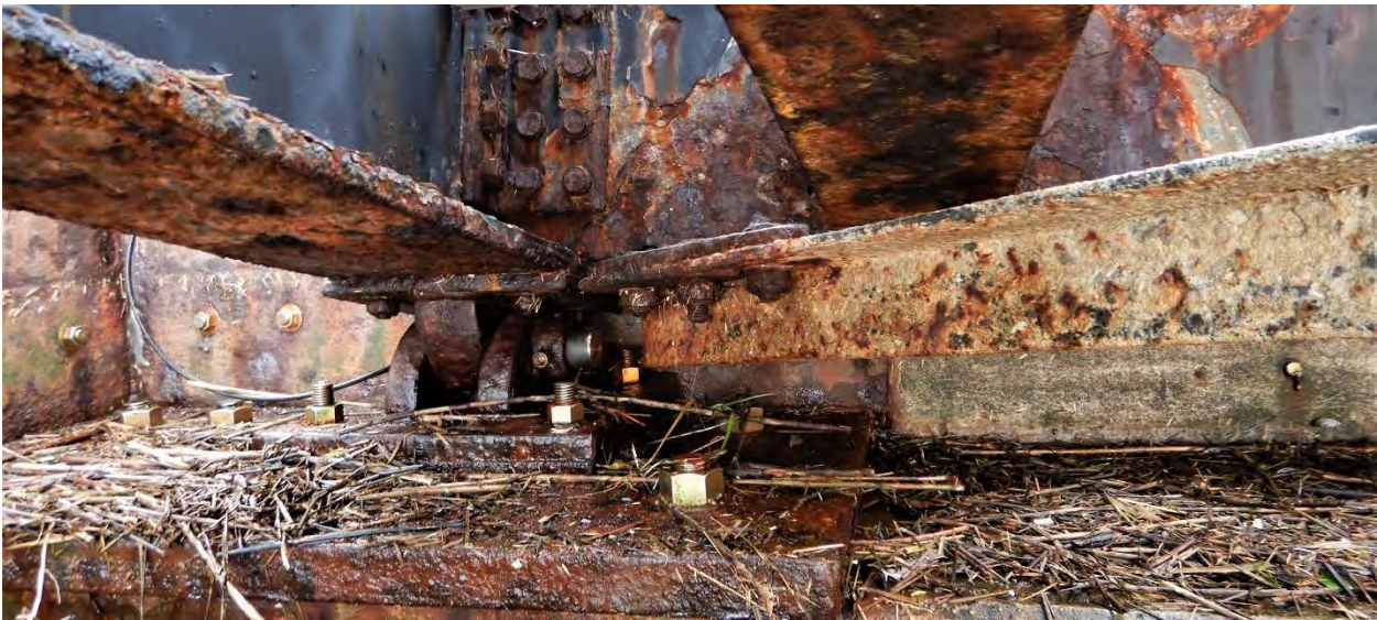
FIGURE 2-21: BHI BARGE RAMP STEEL FRAMING MODERATE CORROSION
