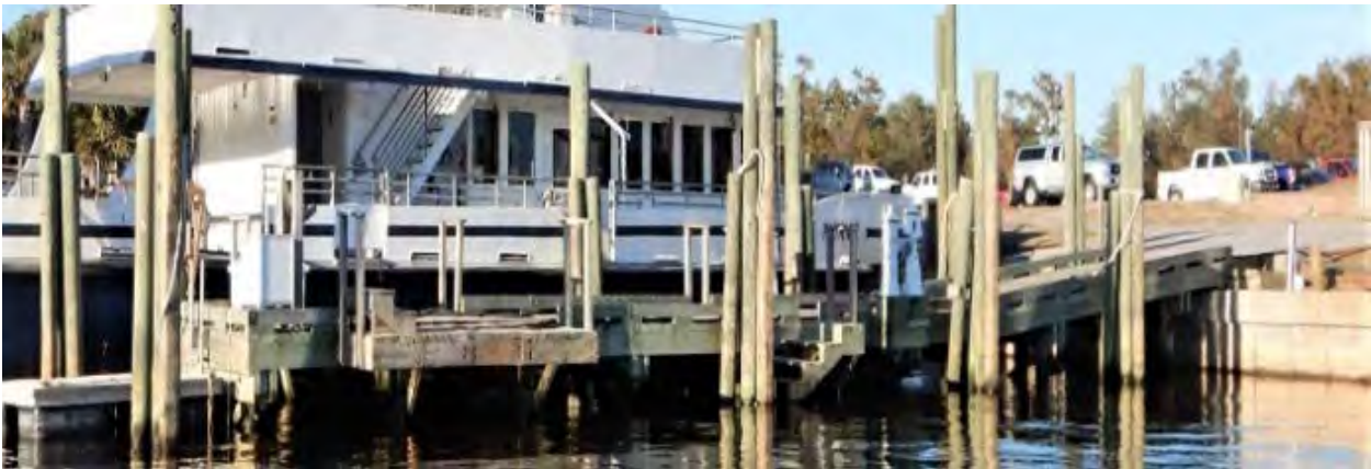
FIGURE 2-6: DPM MAINTENANCE FIXED PIER TIMBER PILE BENTS
