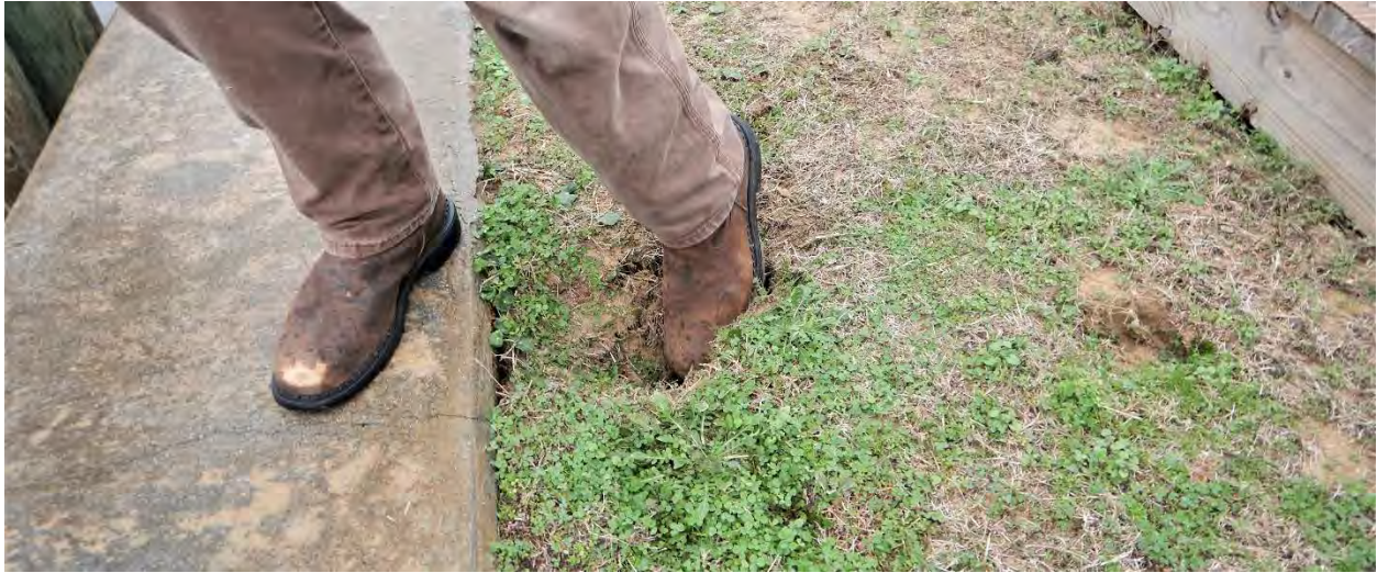
FIGURE 2-15: TYPICAL SINKHOLES BEHIND WALL
