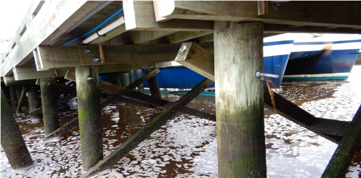
FIGURE 2-6: DPM MAINTENANCE FIXED PIER TIMBER PILE BENTS
